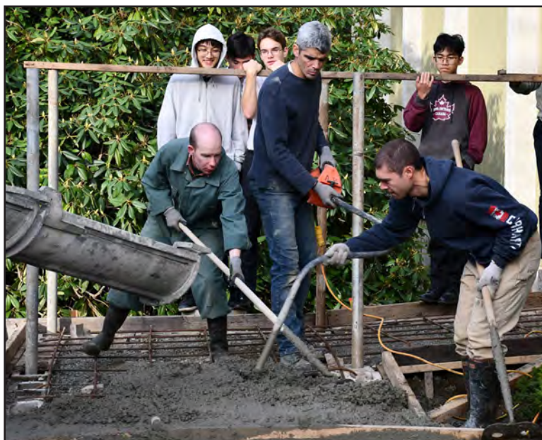
Br Novice Manuel and Postulants Cedric Reimer and Erich Harbich pour concrete for the gym's southwest exit as seminarians observe
